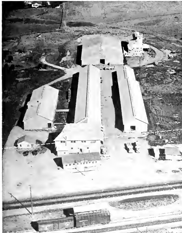
LEFT—Before view. Dotted line shows new right of way boundary. All improvements forward of this had to be relocated. Other lines show former route of trucks to and from loading dock. RIGHT—After view. Dotted lines show where conveyor tunnel lies under freeway. Note relocation of buildings. Mill building has new location. Large new building, upper right, not involved in move.
